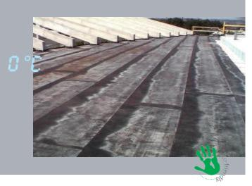
**PROJECT SPECIFICATIONS:** modified bitumen APP membrane particularly suitable for multi-layer solutions in cement, metal or wooden structures, with or without thermal insulation. The versions with HSP polyester are specifically used in applications that require particular mechanical properties (foundations, retaining walls and heavy under-slabs etc.).
